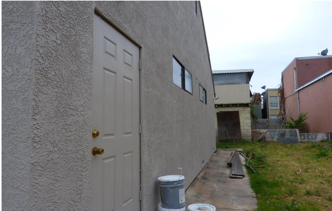
Rear of structure
